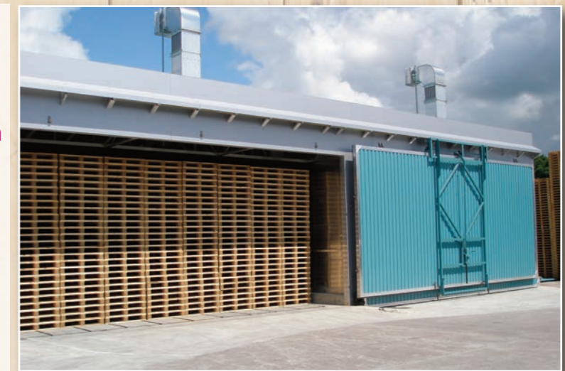
2 Kilns each holding 1225 Euro pallets
