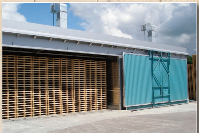
2 Kilns each holding 1225 Euro pallets
